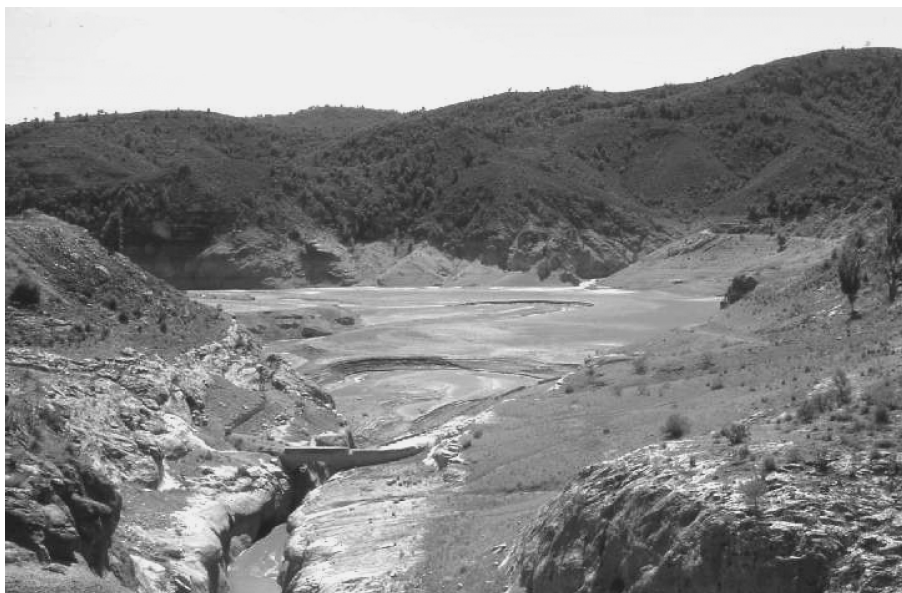
Figure 2.20.1 Sediment deposition in the large La Fuensanta reservoir, SE Spain. According to Avendaño Salas et al. (1997), this reservoir has a storage capacity of 235 \text{ hm}^3 and experiences a mean annual storage capacity loss of about 0.2%. Drainage area equals 979 \text{ km}^2 . (Copyright Gert Verstraeten, with kind permission)
