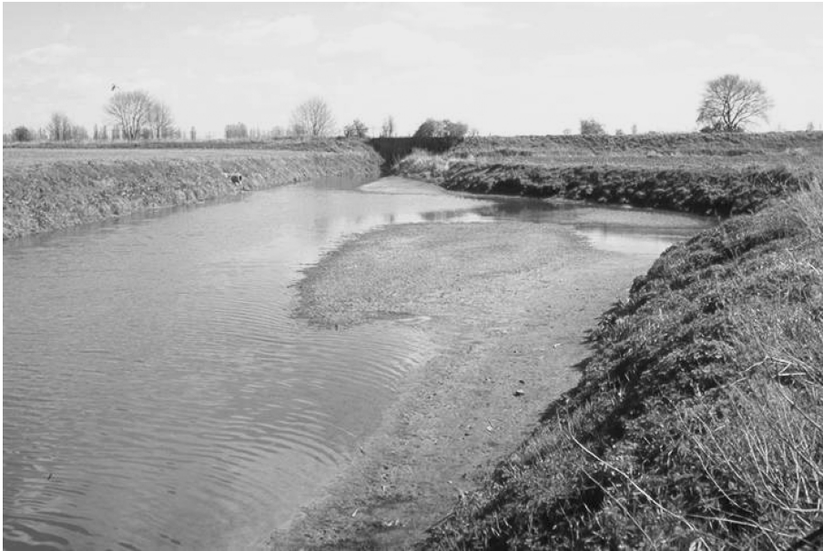
Figure 2.20.2 Sediment deposition in a small flood retention pond in Belgium. It has a storage capacity of 10 000 m 3 and a mean annual storage capacity loss of nearly 10 %. Drainage area equals 48 km 2 (data from Verstraeten, 2000). (Copyright Gert Verstraeten, with kind permission)
